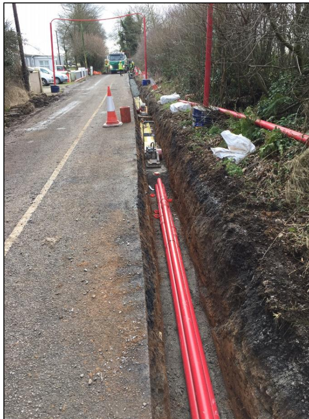
Figure 2.3 Typical UGC Construction
